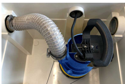
Obr. 16: Montáž AmaDrainer 301 / AmaDrainer 301 C
